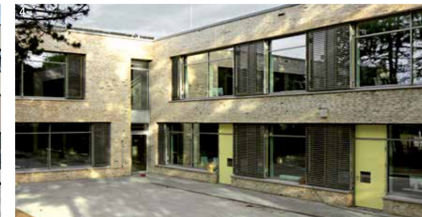
2 + 4 + 6. Extension of the Margarete-Steiff school in Möhringen (GER). Complete service package for 2.300 linear meters of timber-glass façade: planning, material supply, pre-fabrication, transport, and assembly of façade including fix and movable sun protection systems.
